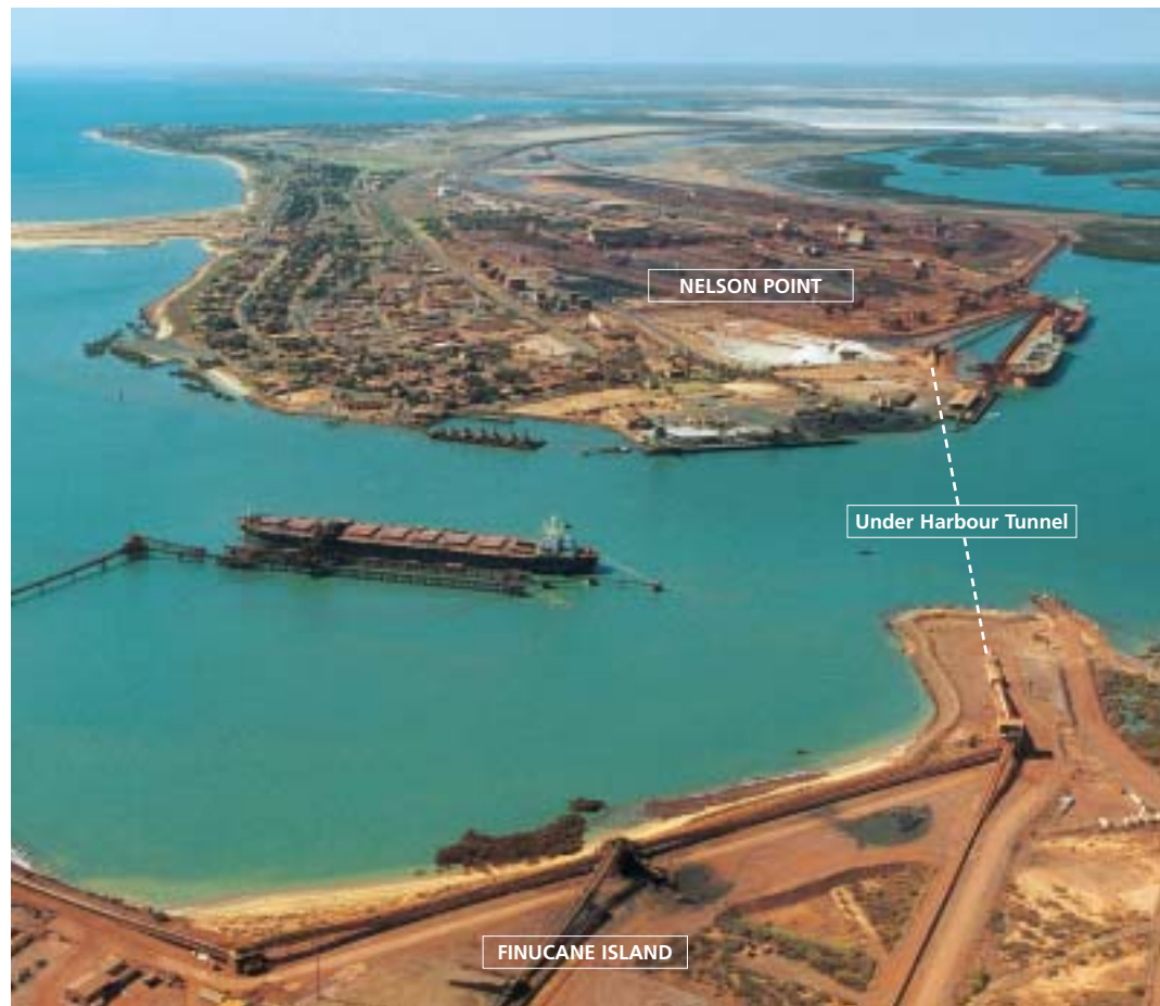
Above Finucane Island and Nelson Point ports, looking from Finucane Island.
