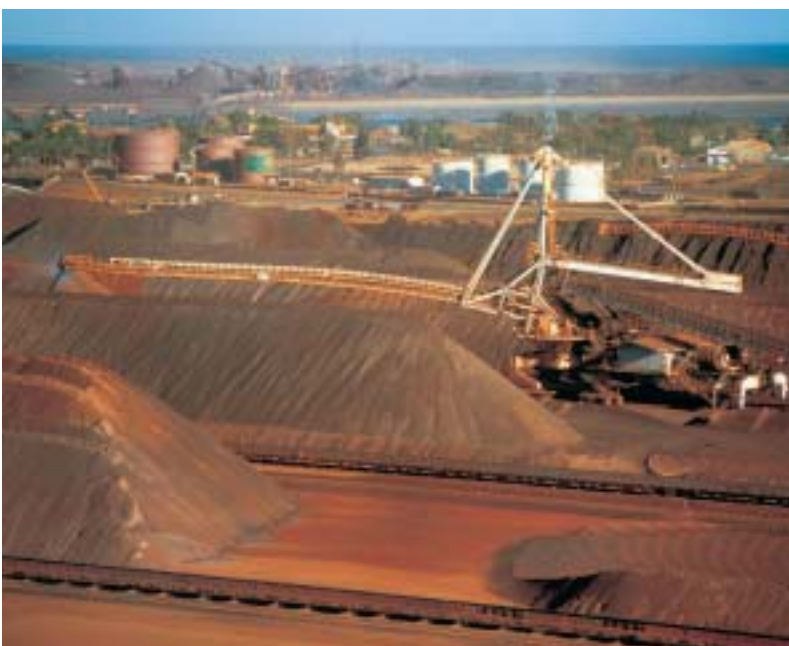
Left A stacker building a chevron stockpile, and in that way homogenising the pile for uniform quality as it stacks.
