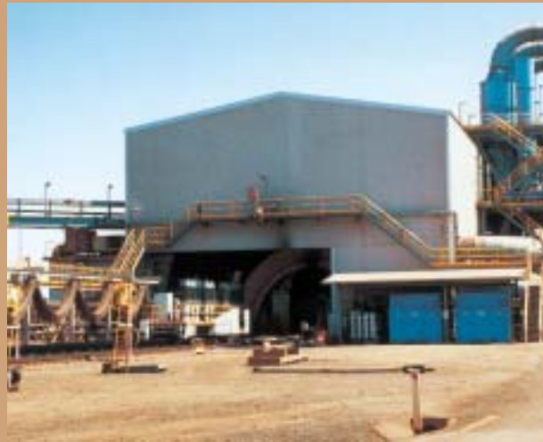
Above Another method of dealing with dust: a large vacuum-extraction system. Rail cars are turned upside-down and dumped in this building.
